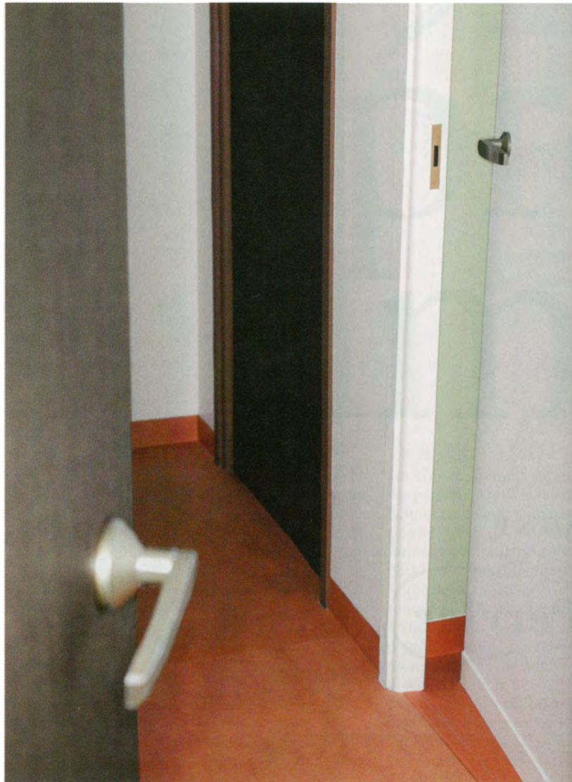
One man's floor is another man's ceiling.
